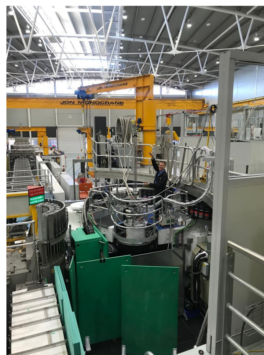
Installation of Triton
